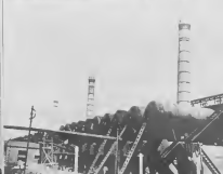
WORKMAN, top photo, seen awoi by this cusher brought by Standard Oil Company of California in February, 1958, a row of high pressure stills, above, at the Baton Rouge Refinery was modern equipment in 1917. At right is a bird's eye view of the refinery, which spread over 540 acres, taken the following year.
